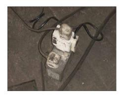
Extension cords and expansion plugs must be plugged directly into the power source without adaptors and should not be used or connected together.
