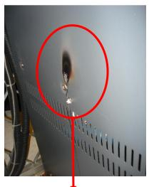
Burnt marks originating from a small fire on the side cabinet of the UPS
