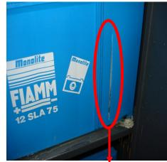
Cracked UPS battery leading to leaking electrolyte
