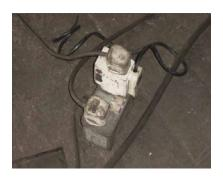
Extension cords and expansion plugs must be plugged directly into the power source without adaptors and should not be used or connected together.
