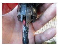
Never use tape to connect or secure electrical fittings, wirings or connections.
