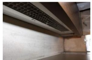
Figure 4 – Front view of vent beside of the toilet bowl where cigarette butts were squeezed through
