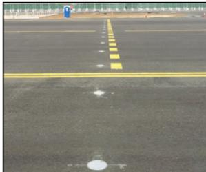
The holding position is a dashed white or yellow line marked across the taxiway, located near taxiway intersections. It is a designated position intended for traffic control at which taxiing aircraft and vehicles shall stop and hold until further cleared to proceed by air traffic control. When instructed to hold short of a taxiway ahead, drivers shall come to a complete stop before this line.
