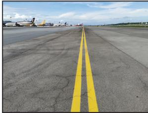
The taxiway edge line is a pair of continuous yellow lines that mark the edge of the taxiway. Near turns, 90-degree notches extend from the edge lines toward the taxiway shoulder.
