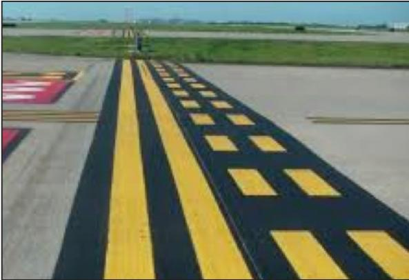
Runway holding position markings contain two solid and two dashed yellow lines across the width of the taxiway. The solid side is closer to the taxiway, while the dashed side is closer to the runway.
