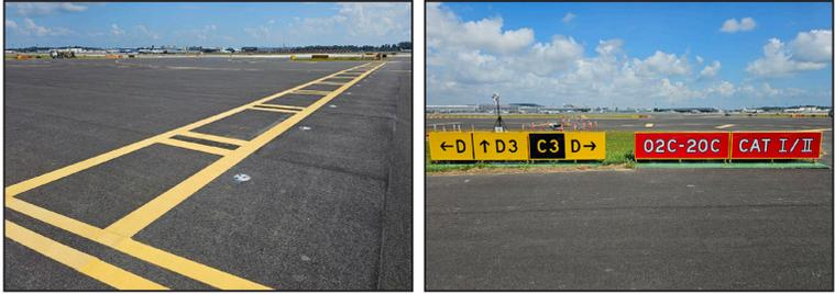
The CSA east of Runway 2 overlaps with taxiways D12 through D14 and C12 through C14 at Runway 2 South, and taxiways D1 through D3 and C1 through C3 at Runway 2 North. These 2 zones are protected by ladder markings; mandatory signs; microwave barrier detectors (MBD), and red stopbars. The stopbars are turned on whenever the corresponding runway direction is in use (for example, when 02C is in use, the stopbars at the south end will be turned on, while the stopbars at the north end will be off).
