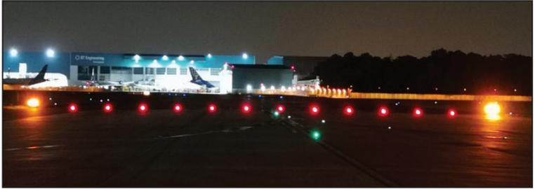
Runway holding positions are accompanied by steady red stopbar lights and alternating flashing amber runway guard lights.
