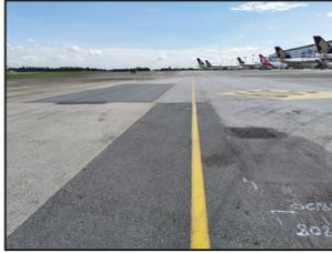
The taxiway centerline is a continuous yellow line that marks the center of a taxiway. Generally, drivers should drive along the taxiway centerline to help stay on course and to provide the largest field of view from both sides of the vehicle.
