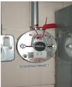
Activate the kitchen fire suppression system manual pull switch if the fire is cannot be extinguished using portable fire extinguishers. Do not use water on cooking oil fires.
